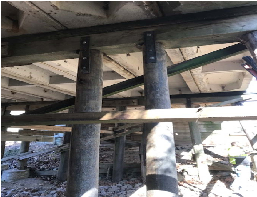
REPAIRED PILES "G" & "H" IN BENT #1
