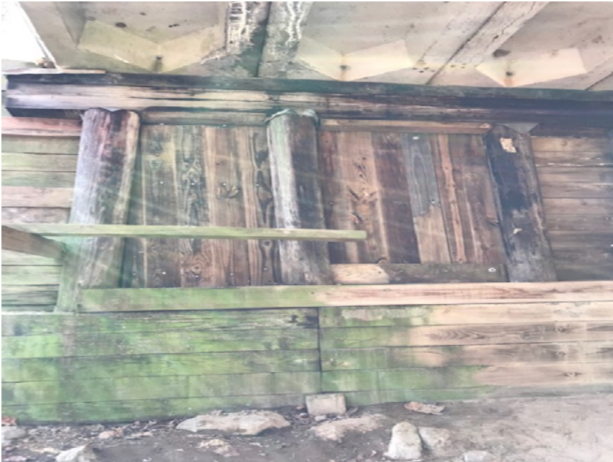
REPAIRED PILES "G" & "H" IN BENT #1
