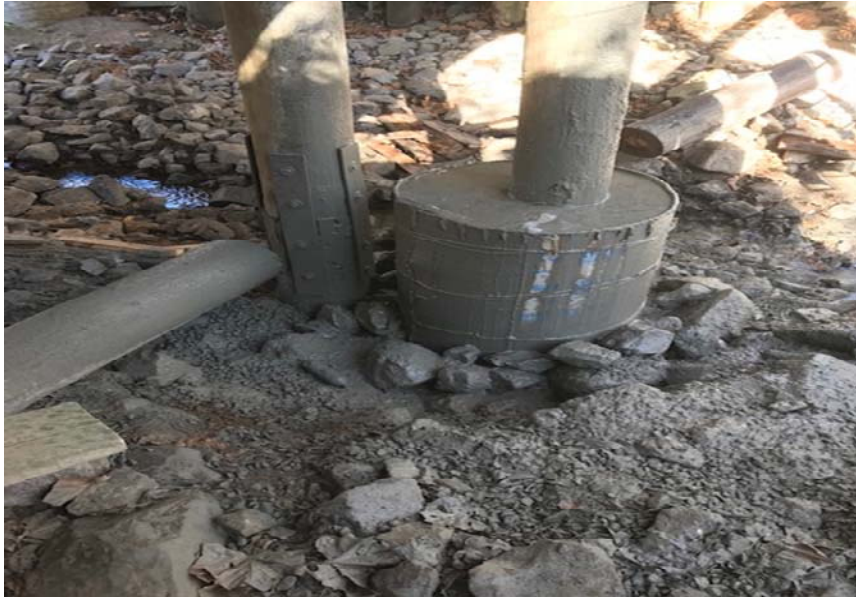
REPAIRED PILES "G" & "H" IN BENT #1
