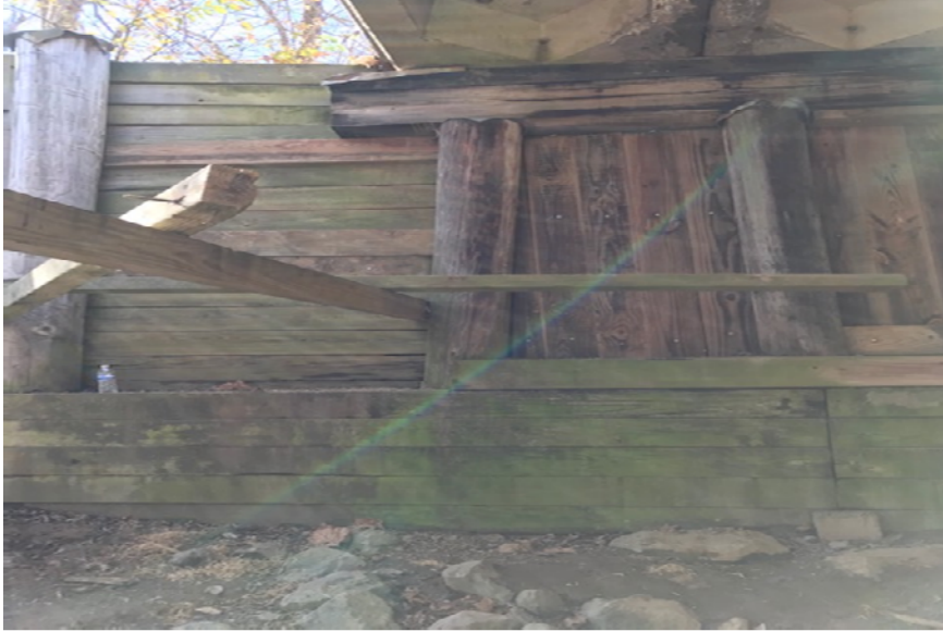
REPAIRED BREASTWALL & WING AT ABUTMENT #1 & BREASTWALL AT ABUTMENT #2
