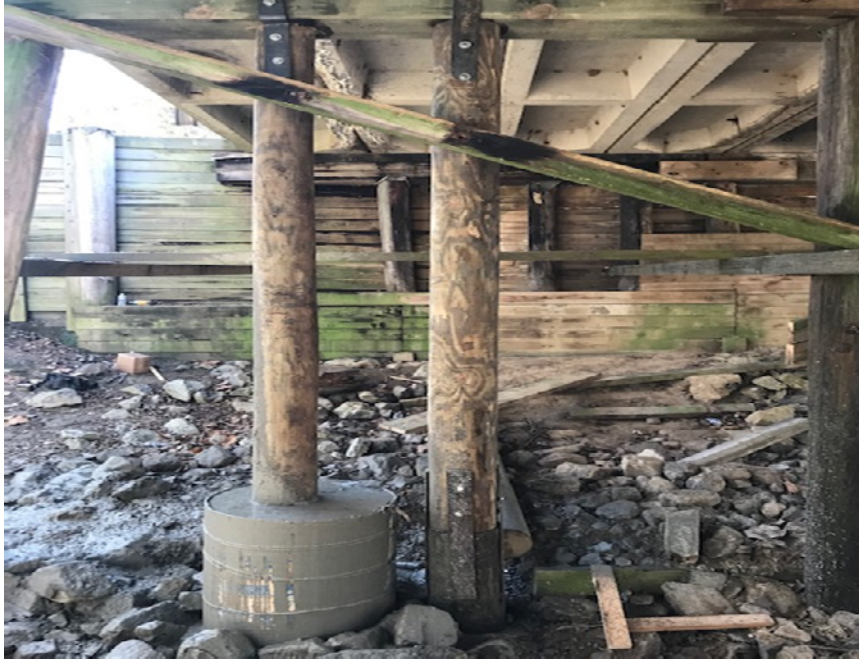
REPAIRED PILES "G" & "H" IN BENT #1
