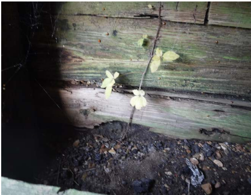
ABUTMENT # 1 BREAST BOARD DECAYED
