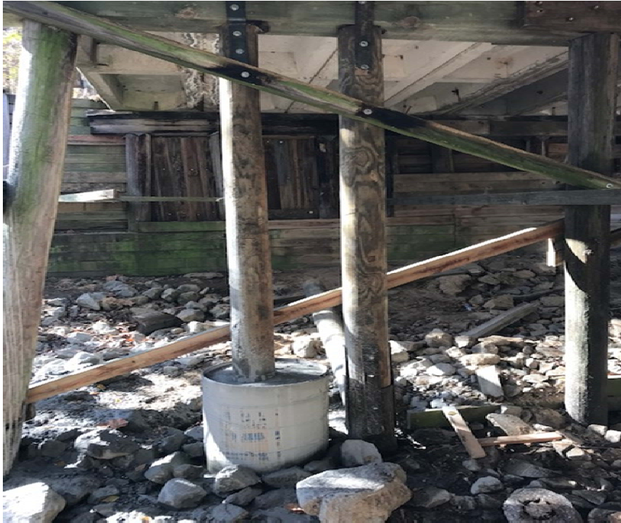
REPAIRED PILES "G" & "H" IN BENT #1
