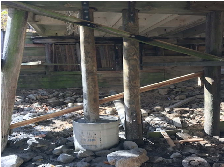
REPAIRED PILES "G" & "H" IN BENT #1
