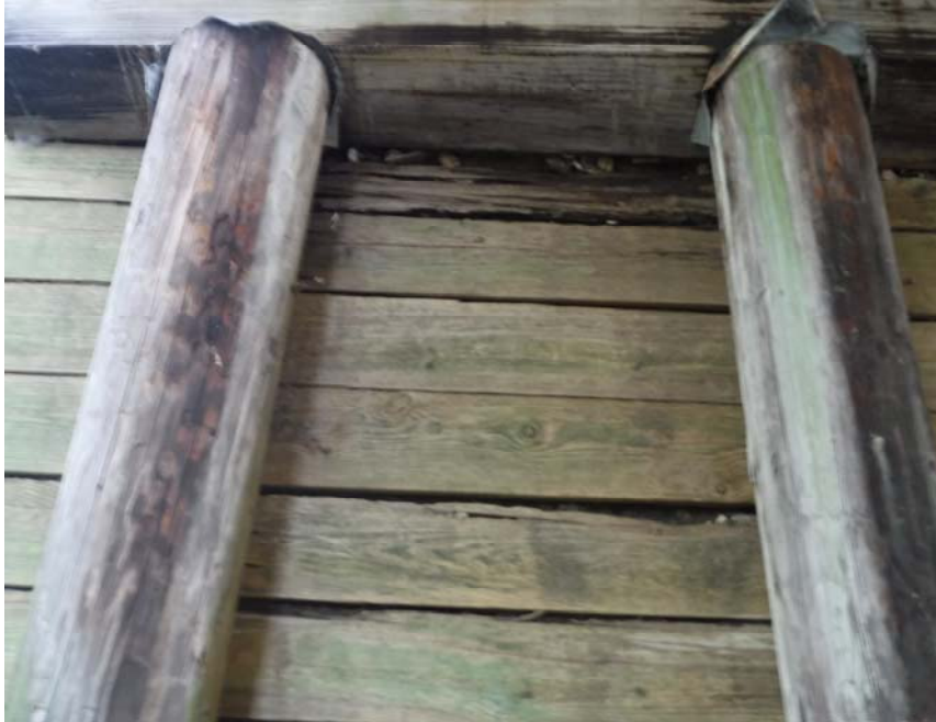
ABUTMENT # 1 BREAST BOARD DECAYED
