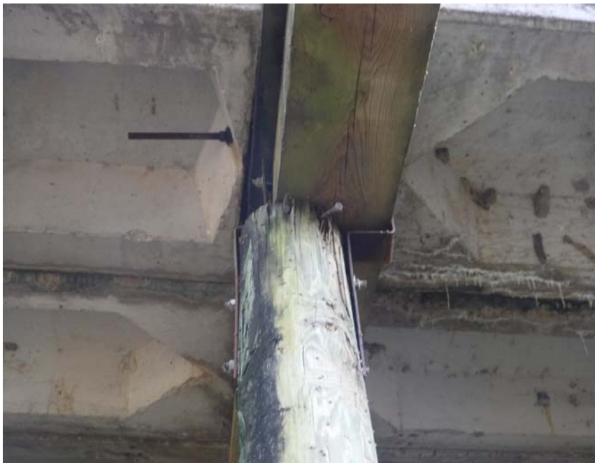
SPAN # 1 SLAB "B" SPALL TO STEEL
