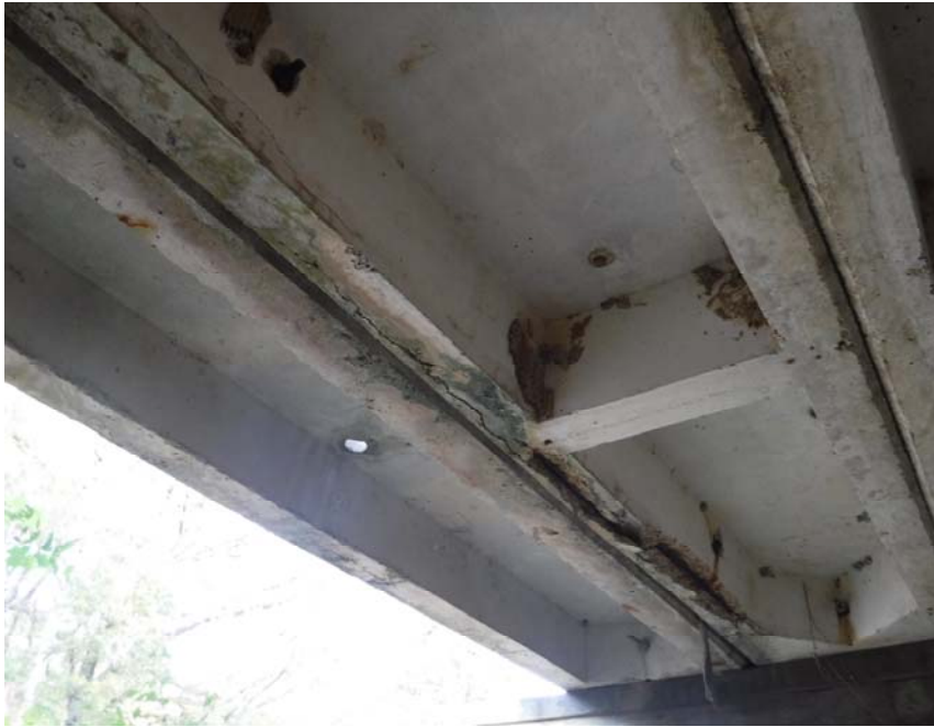
SPAN # 1 SLAB "B" SPALL TO STEEL
